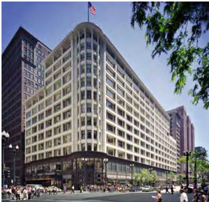
View of Carson, Pirie, Scott and Co. (now the Sullivan Center) in 2007. The building, one of the most famous early skyscrapers, was designed by architect Louis Sullivan in 1903 and is now a National Historic Landmark.
